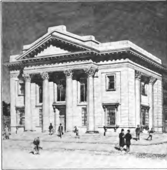
THE BANK BUILDING.
